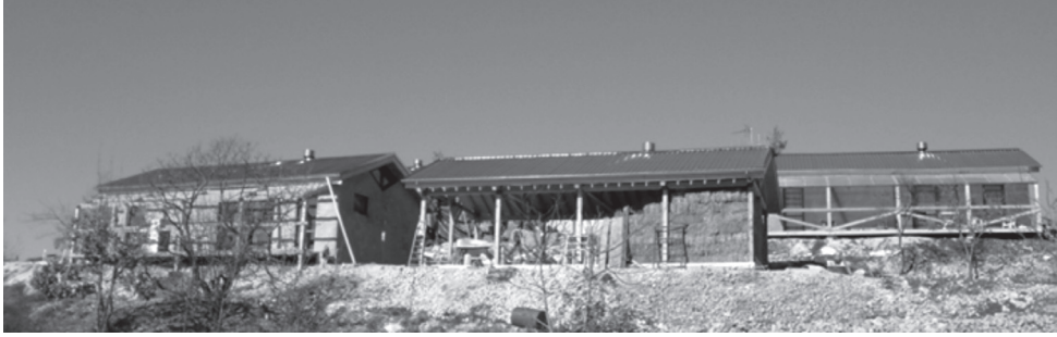
Figure 2 EVA construction in progress, 12 February 2011
